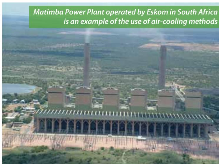
*Matimba Power Plant operated by Eskom in South Africa is an example of the use of air-cooling methods*
